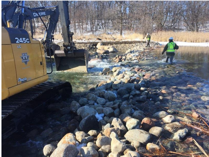
Setting weir 1 with help of DNR
